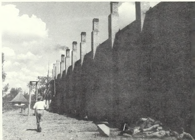
Southern Rhodesia: Flue-curing barns are built in blocks of four, six, eight, or more. Fuel may be wood, coal, paraffin
